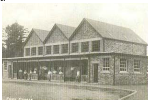
Rugby Fives Courts, built Spring 1934
